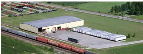
Stevens Rail Facility Teutopolis, IL
