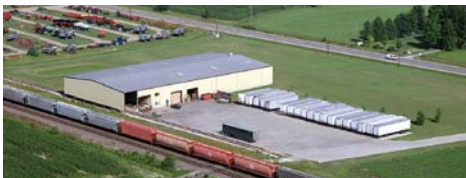
Stevens Rail Facility Teutopolis, IL
