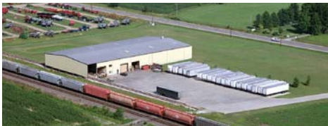
Stevens Rail Facility Teutopolis, IL
